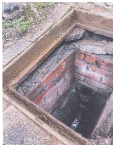
P1 10 MH Frame and Pavicours lifted.
