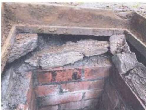
P 9 Root just visible in top LH corner of MH Frame.
